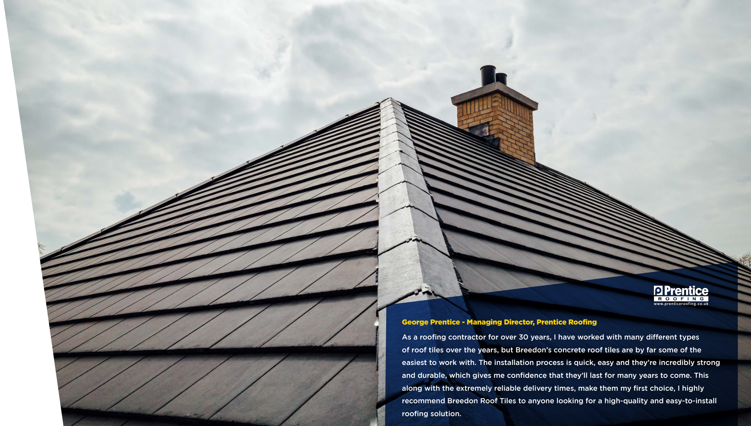
UNIVERSAL ANGLE HIP BLOCKEND Length 455mm Also available to suit Third Round and Elite
